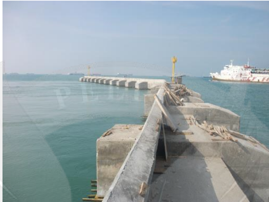
Gambar 1.1 Breakwater Pelabuhan Merak (Sumber: P.T. Cemerlang Samudra Kontrindo)
